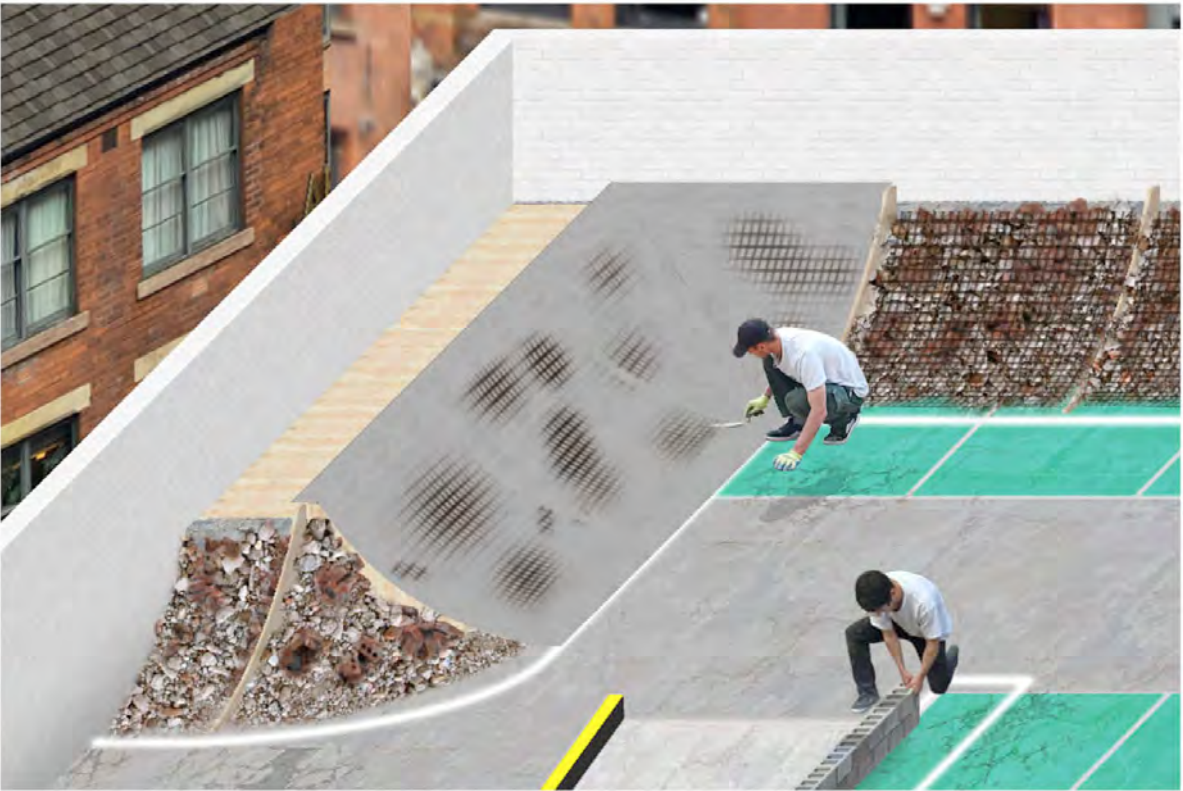
6 - Cover with cement concrete and scrape smooth when semi-dry
