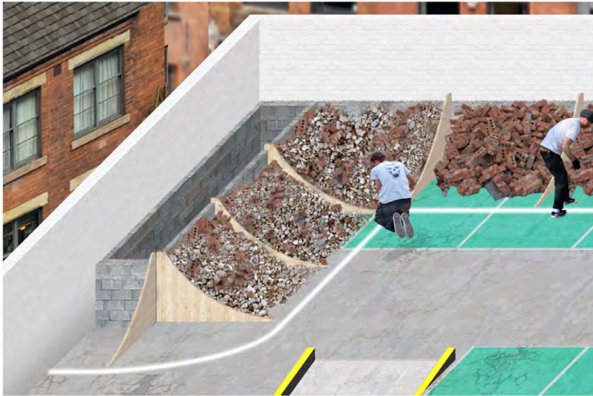
4 - Cover fill with finer gravel/aggregate
