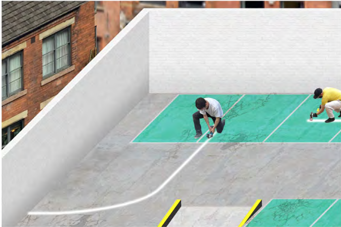
1 - Mark out footprint but cutting into floor
